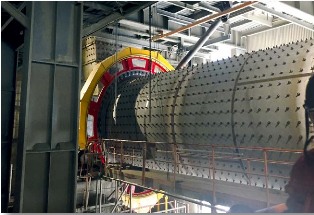
Figure 5: SEW girth gear with protective cover (Photo: Cemex)
